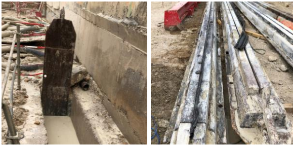
Fig. 13. CWS formwork for D-Wall panel joints.
