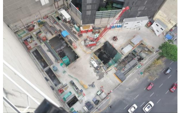
Fig. 25. Top-Down excavation works for 8 basements.
