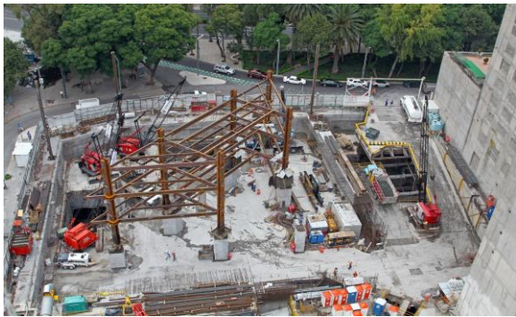
Fig. 23. Simultaneous construction of superstructure.
