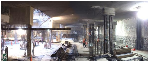
Fig. 23. Simultaneous construction of superstructure.
