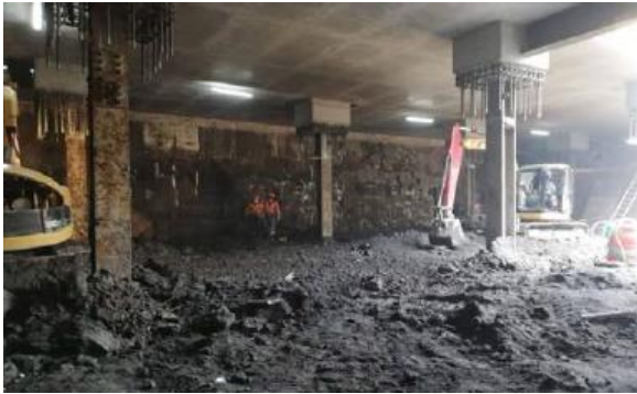
Fig. 9. Definitive columns built while excavating.
