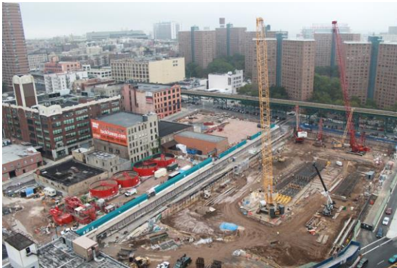
Fig. 28. D-Wall and Pile works for Top-Down.
