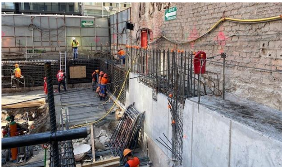
Fig. 18. Size and reinforcing of a D-Wall capping beam.
