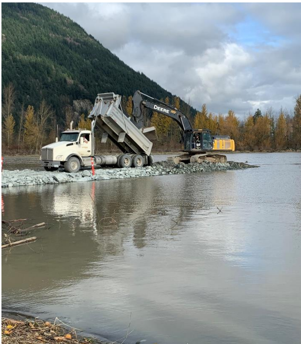
Fig 5. Initial Breach Closure.
