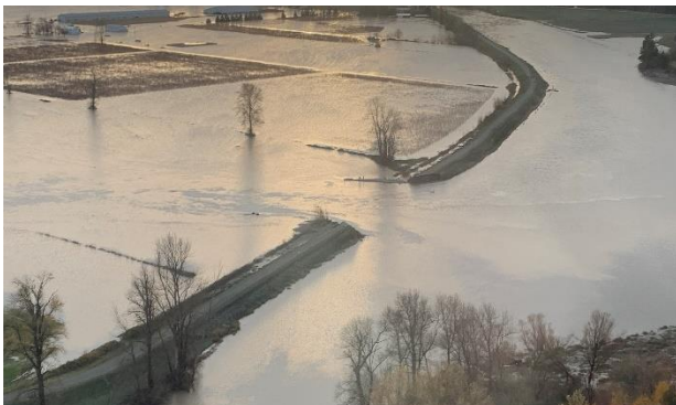
Fig 3. Aerial image of the dike breach.
