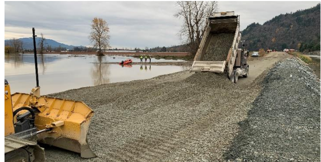
Fig 6. Construction of the breach closure.
