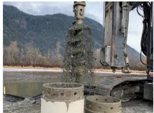
Fig 14. Pre-drilling with casing.
