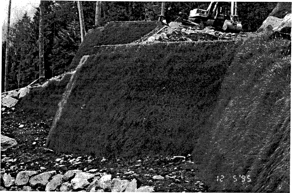
Figure 9 - 4 m high wall 1 month after completion
