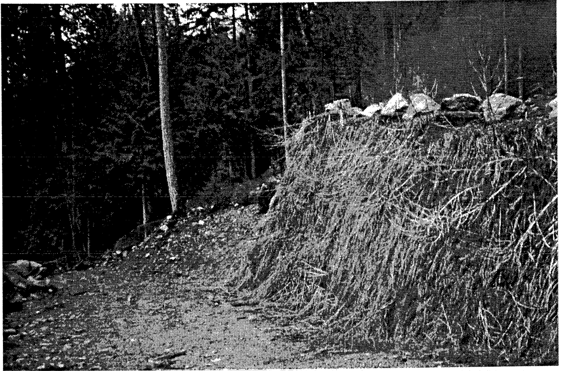
Figure 11 - 1 year after construction
