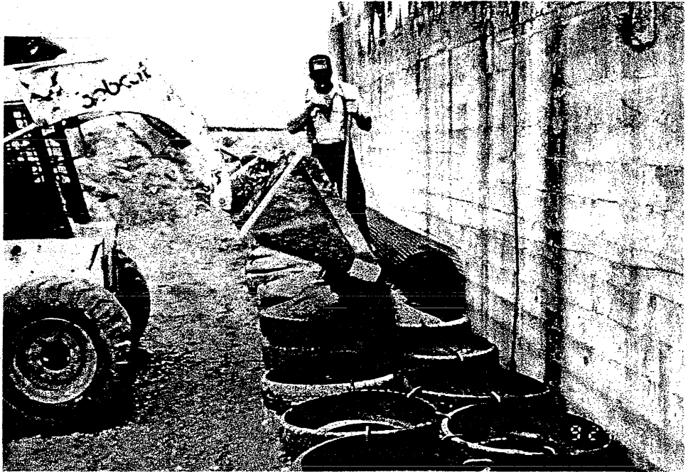
Figure 10: Typical tire backfill process
