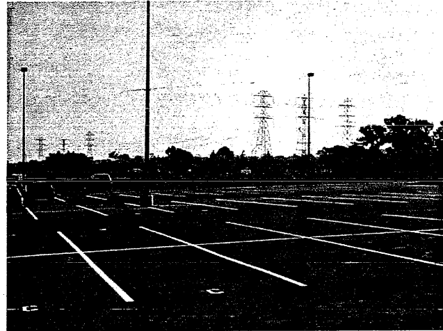
Fig. 3. Asphalt surfaced parking areas are an economically attractive land use for construction above landfills for park and ride facilities.
