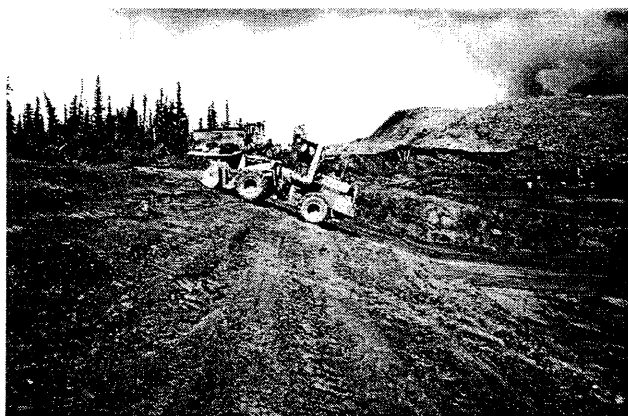
Fig. 2. Preparing Subgrade by Backblading with Front End Loader
