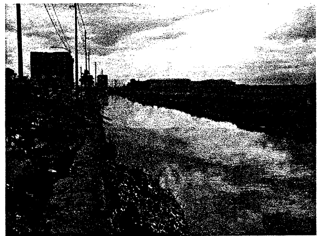
Photo 1. View South Along Canal. Coastal Mall is in the Background
