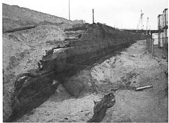
Fig. 9. Wire facing with P300 turf reinforcement
