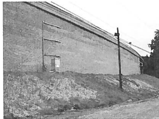
Figure 3. Wall C as completed.
