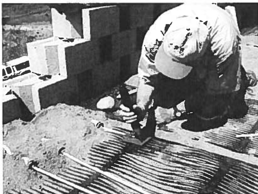
Figure 2. Installation of extensometers.
