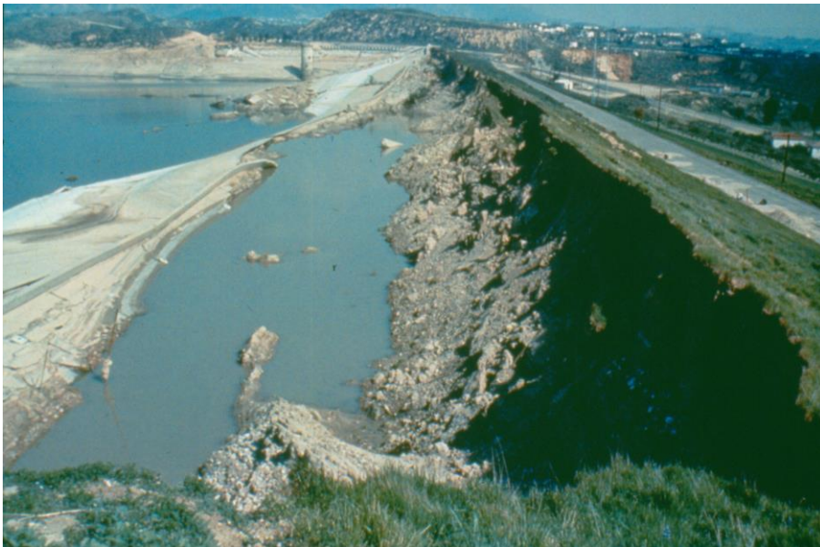
Lower San Fernando Dam in 1971 (DSOD files)
