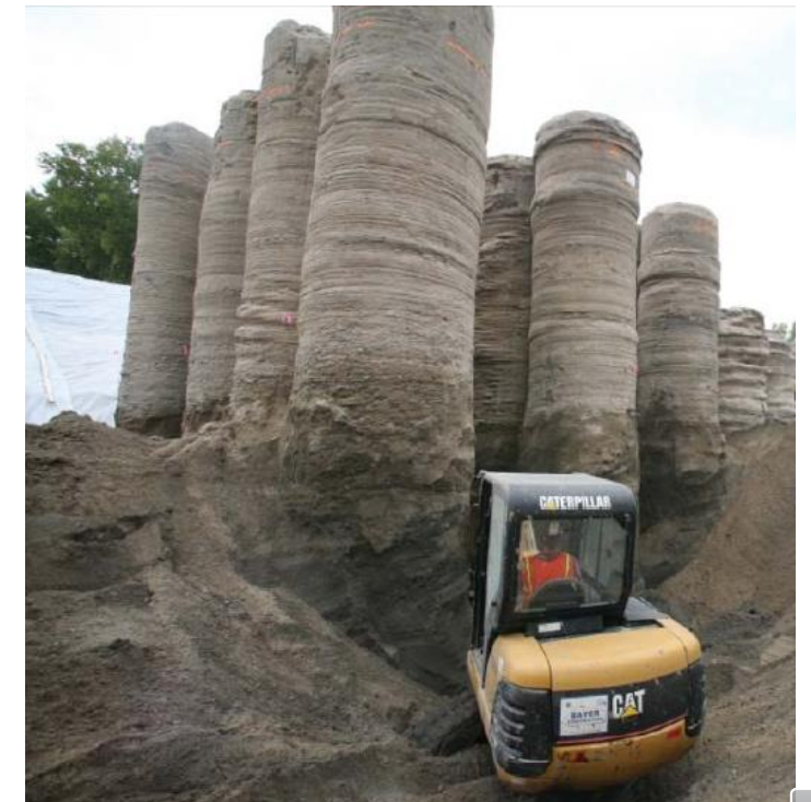
Jet grout columns (John Dillon 2009)
